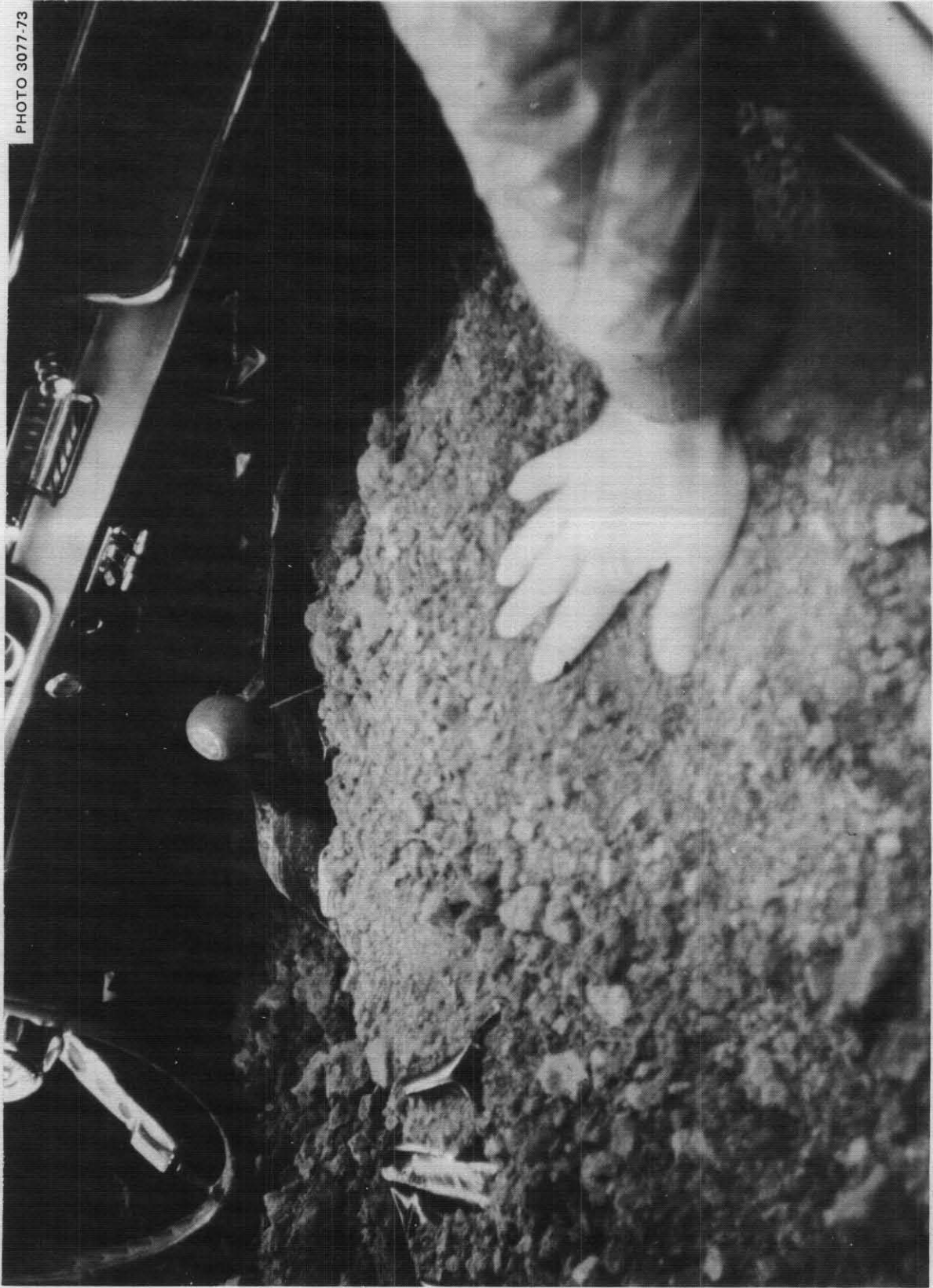
Fig. 6.11. About a foot of earth inside the car. Note the black plastic lining under the earth. Kearny, after several families had refused his offer of $250 to build a Car-Over-Trench Shelter in 36 hours or less, offered to supply the car-protecting plastic.
